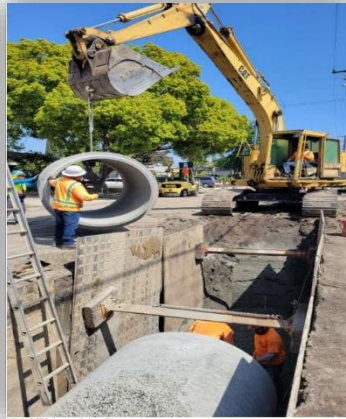
The Acacia-Josephine Storm Drain in construction.
