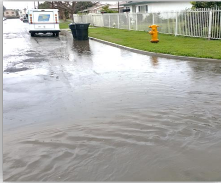
Flooding in the Acacia-Josephine Neighborhood during the rainy season before construction of the storm drain.
