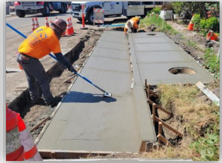
The Acacia-Josephine Storm Drain in construction.
