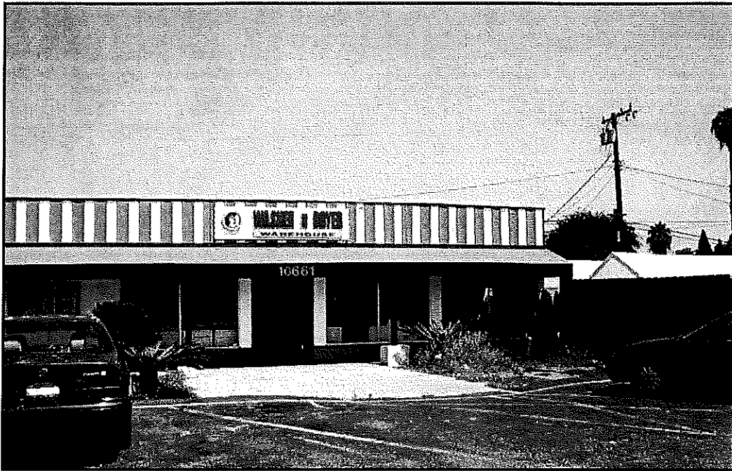
View of existing business along the Garden Grove Blvd. frontage (10661 Garden Grove Blvd.). This building will be demolished to accommodate the project.
