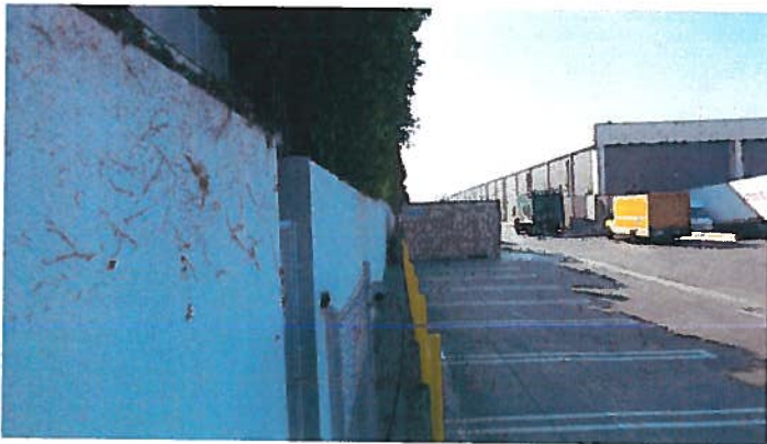
Noise Measurement Site 2 - Looking south
