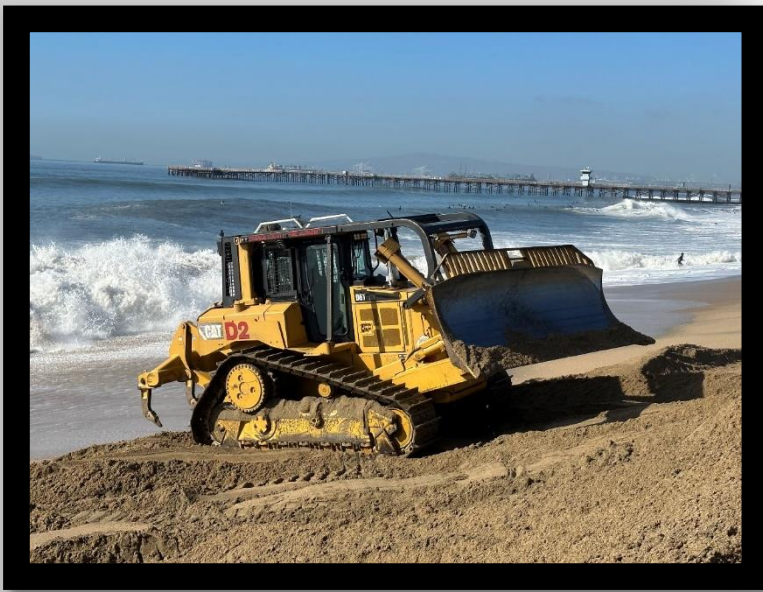
Heavy Equipment Operators building sand berms in Seal Beach.
