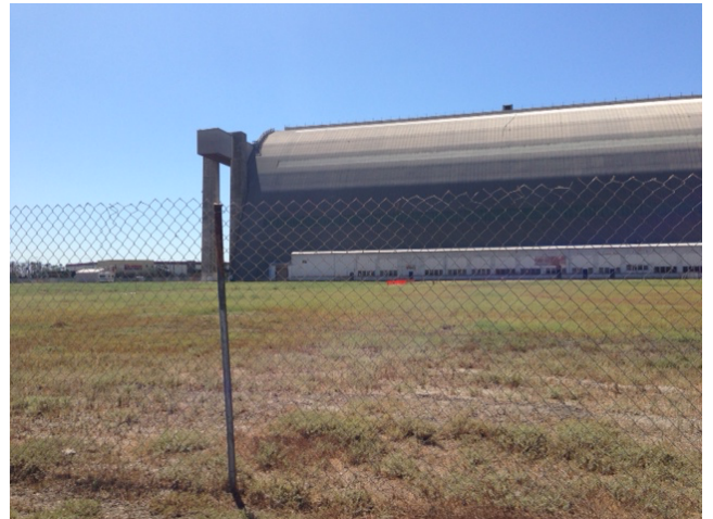
South end of the north hangar in 2015. This is the closest I could get!
